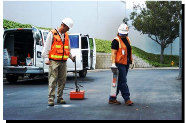
Ground Penetrating Radar and 50/60HZ
